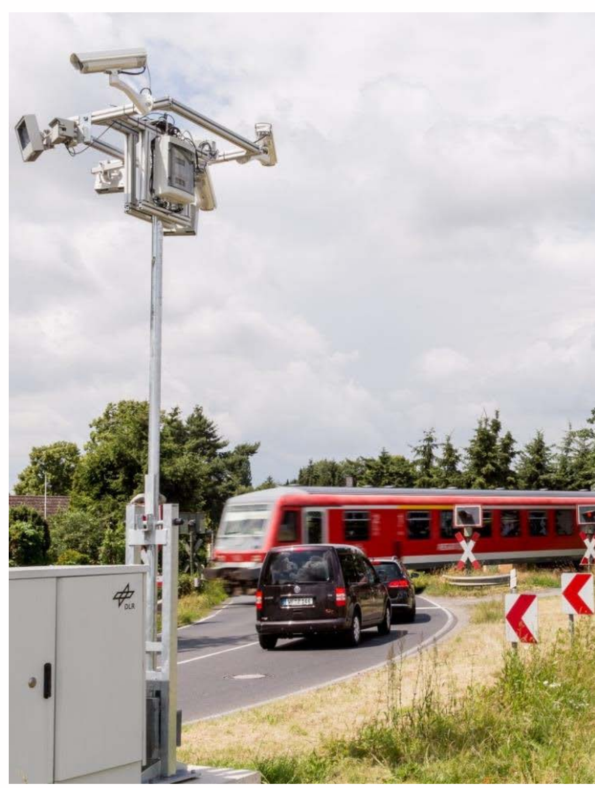
Measurement campaign at a level crossing with a flashing signal
